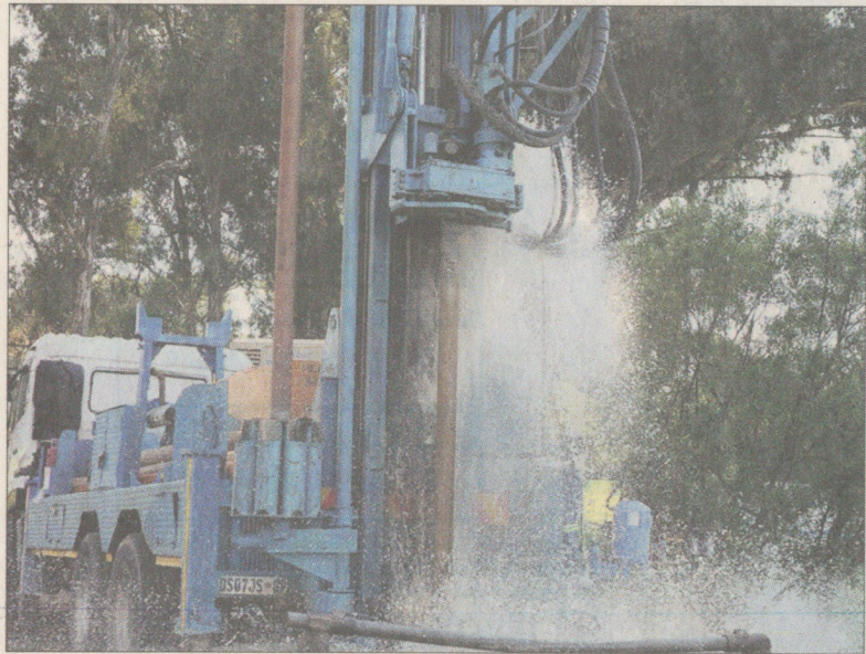
WET GOLD: A drill rig bores a 70m borehole which will provide the Bryanston Country Club with water.
