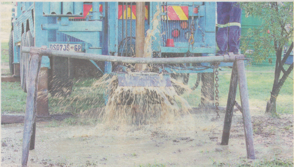
The borehole water demonstration shows the sheer force of the water.
